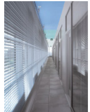
This "loggia" acts as climatic regulator for each floor.
